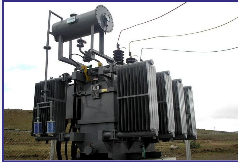
Converter And Rectifier Transformer
